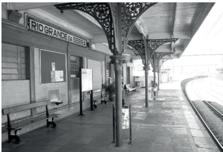
Figure 1 – Rio Grande da Serra railway station. Source: Field research – III Steamcon. Author’s file. Photograph: Gilson Pedroza.
